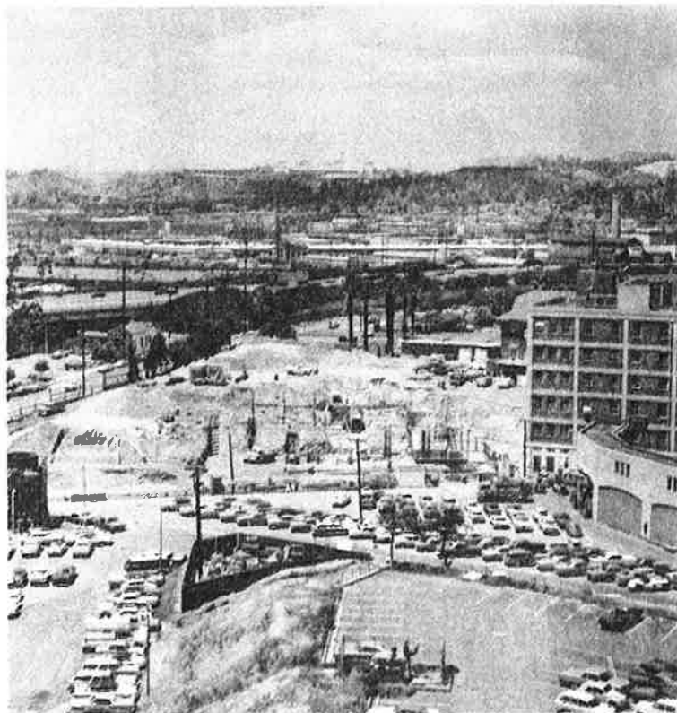
Photograph taken April 27, 1970 showing building construction
