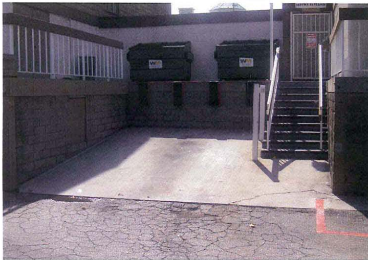
7- SERVICE/LOADING DOCK OFF ALLEY
