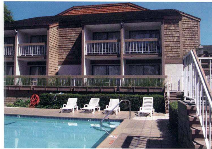
18- BLDG. B FROM POOL DECK
