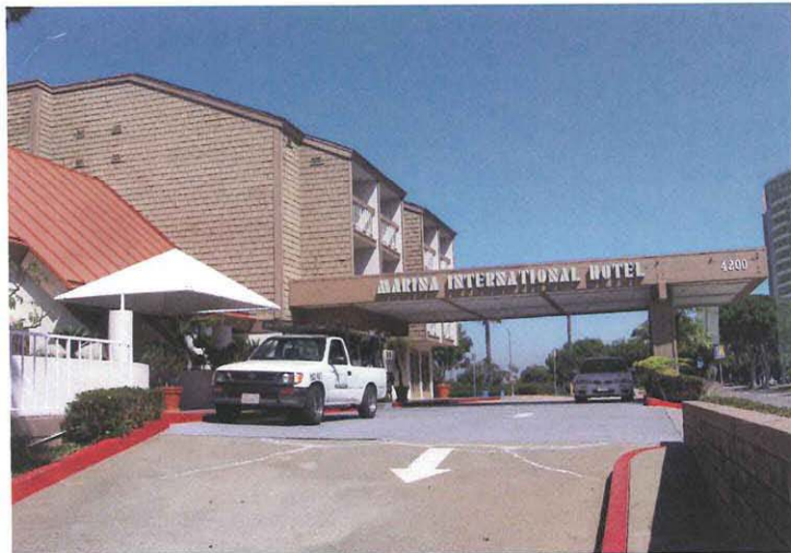
3- HOTEL ENTRY FROM RAMP DOWN TO PARKING
