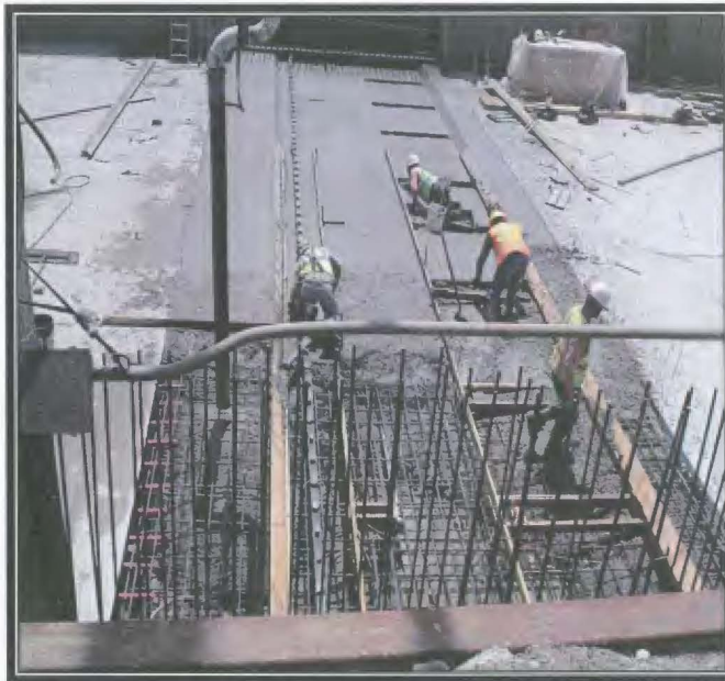
Construction of the new Rubber Dam at Hansen Spreading Ground.
