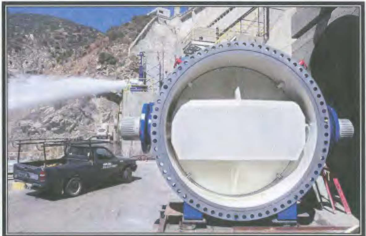
A 96-inch Butterfly Valve is being prepared to be moved into the valve chamber inside Morris Dam.
