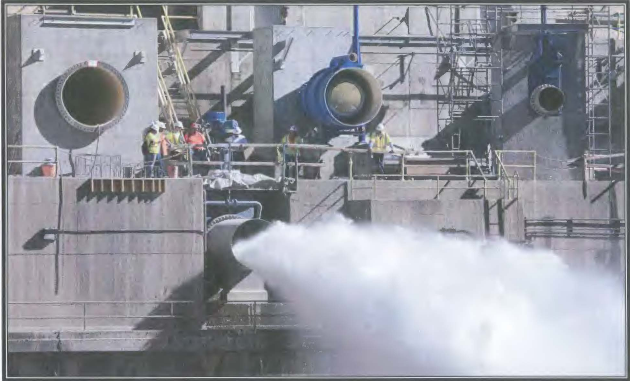
Testing the new 40-inch Jet Flow Gate Valve.
